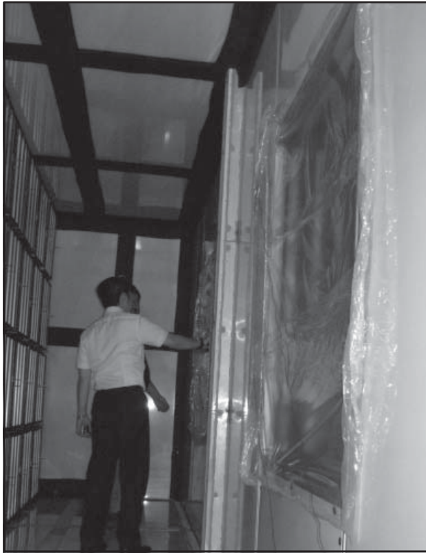
FIGURE 1. HVAC Main Supply
