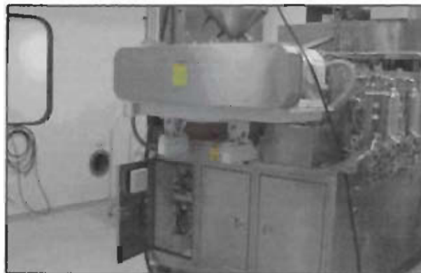
Figure 1. Room housing an operating BFS machine
